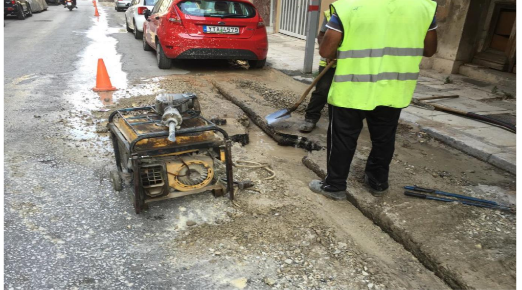
Water pipes not in the street plans or not as deep as expected
