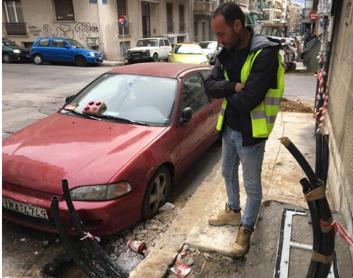
Abandoned cars where you want to dig
