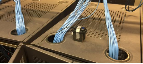
Fig. 2: Inertial measurement unit (IMU) on top of a DC rack.
